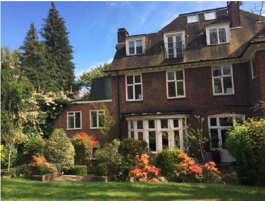
Photo 2- Rear elevation showing existing side extension
