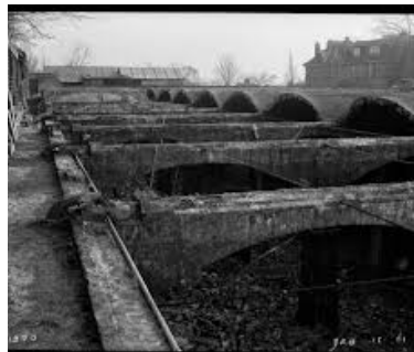
Kidderpore Reservoir - Thames Water archive.thameswater.co.uk
