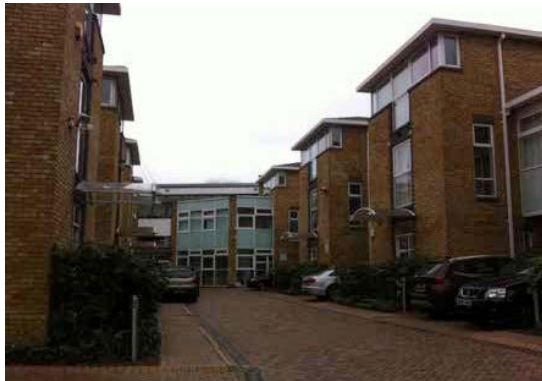
Photo 22: Hampstead Gate, Internal Site Streetscape
