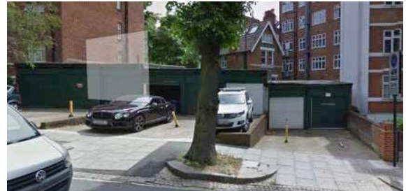
Photo 20: Frognal Lane Garages, Streetscape
