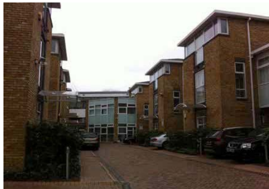
Photo 22: Hampstead Gate, Internal Site Streetscape
