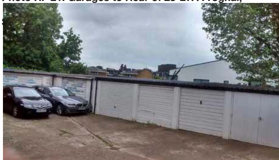
Photo RF 21: Garages to Rear of 23-27A Frognal,
