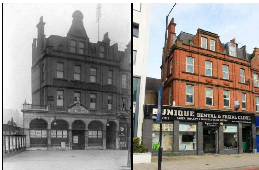
Photo14: Original and Existing Shopfronts at 200 Finchley Road
