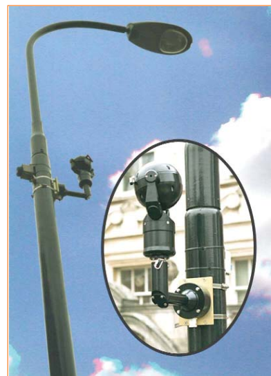
‘Metal Mickie’ camera on a lighting column
