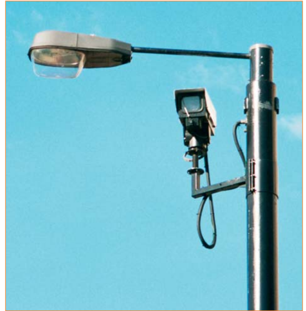
Combined CCTV and lighting column
