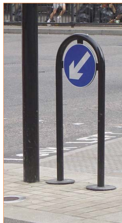
Externally illuminated metal hoop ‘keep left’ sign
