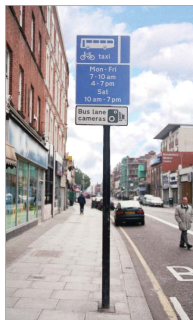
Separated signs carefully aligned on a post
