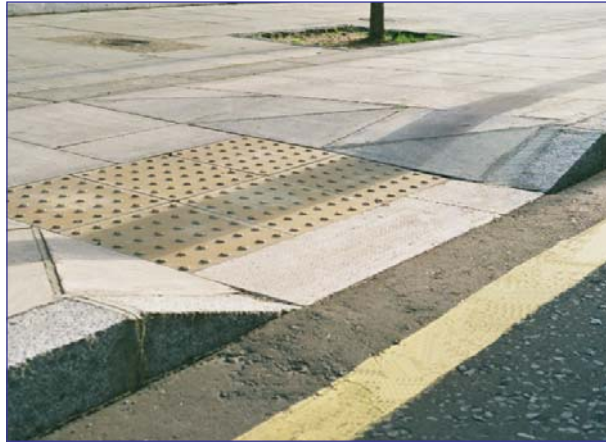
Details of dropped kerbing in John St
