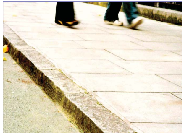
Boulevard paving laid with 150mm staggered bond
