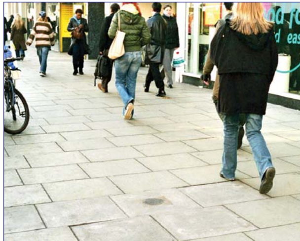
Boulevard paving on a busy commercial street
