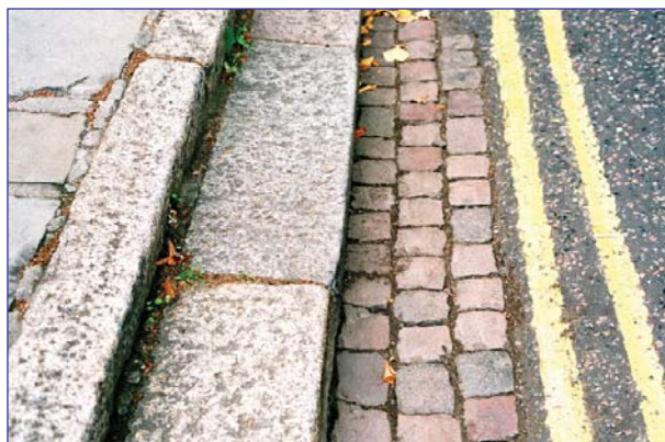
Double granite kerb with drainage channel
