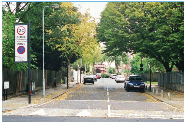
Raised entry treatment in St Cuthberts Road
