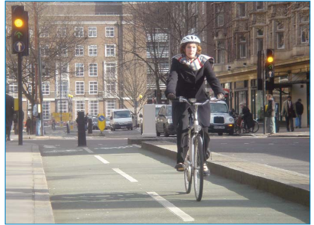
Segregated cycle lane in Torrington Place
