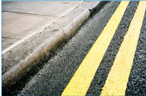
Canary yellow lines at 100mm width
