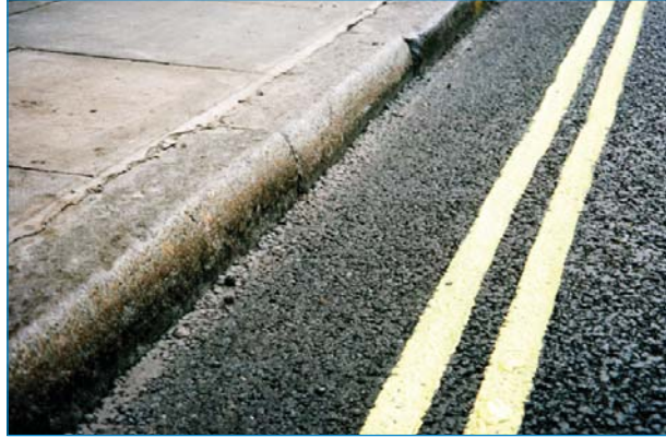
Primrose yellow lines at 50mm width
