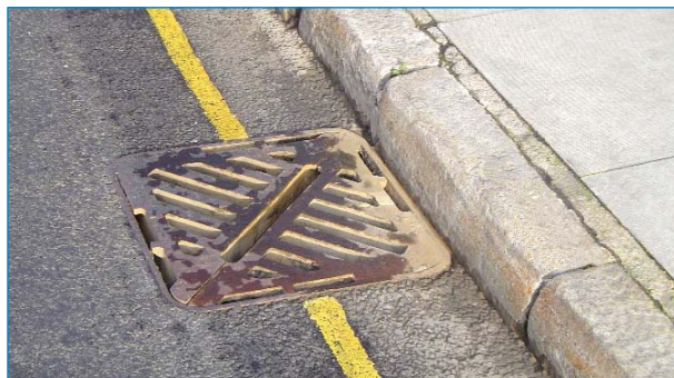
Carriageway gully cover – Double triangular D400
