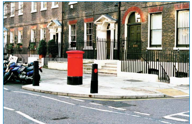
Footway build-out in John Street
