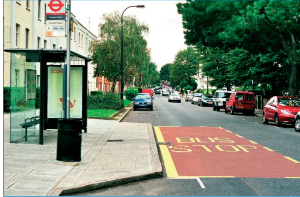
Bus boarder in Belsize Road
