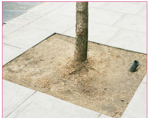
Tree pit in footway with water pipe
