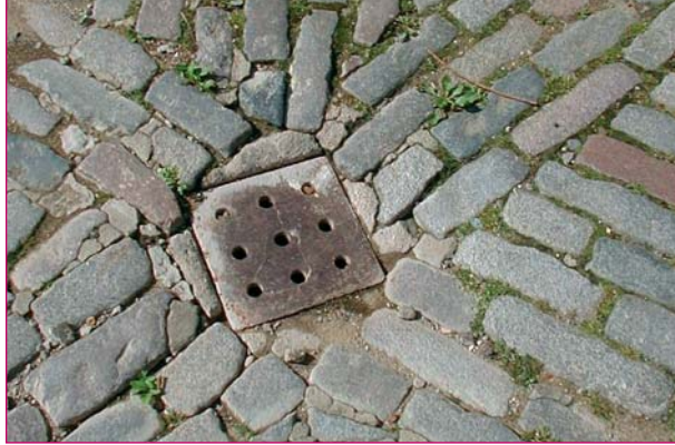
Setts used in traditional drainage techniques
