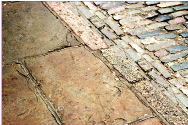
York stone and old granite setts
