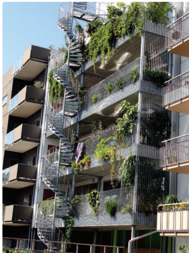
Fig. 7 In the 'Urbana Villor' project the large balconies have 300 millimetre substrate covering the whole balcony area. A system of tiles makes it possible to use as little or as much as one wishes for vegetation, but the roots have large volumes of substrate. The balconies are not attached to the wall, but to a free-standing structure to avoid humidity problems
