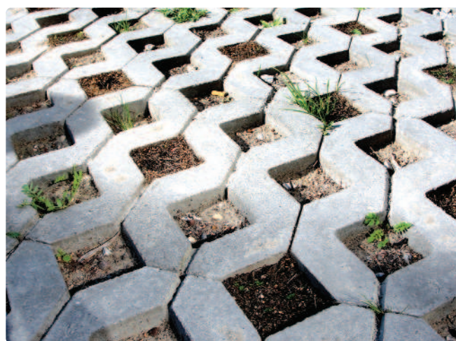
Fig. 8 One of the courtyards at Flagghusen, Western Harbour, Malmö, is to a large extent built with permeable concrete blocks. The permeability helps in reaching the required Green Space Factor, but most people would agree that the courtyard has low aesthetic value
