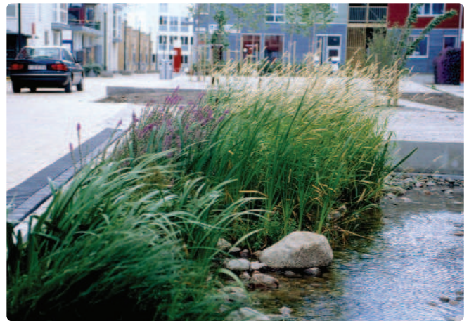
Fig. 1 Vegetated ponds form an important part of the stormwater system at Bo01, Western Harbour, Malmö
