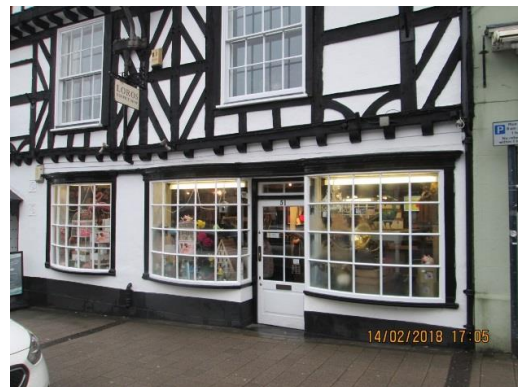
51 Market Street, Ashby. Black gives visual 'strength' to the main frame elements but white has been used to pick out other elements. The use of black and white respects the finishes of the building.
