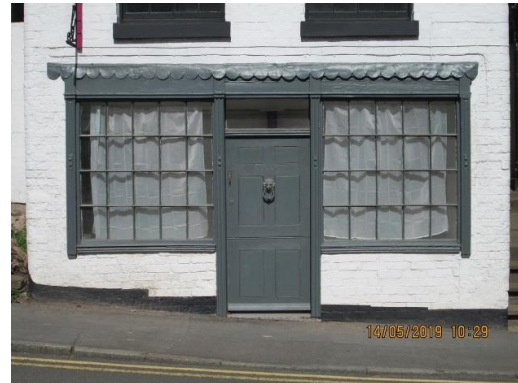
89 Bondgate, Castle Donington. Mid nineteenth century; note the small panes.
