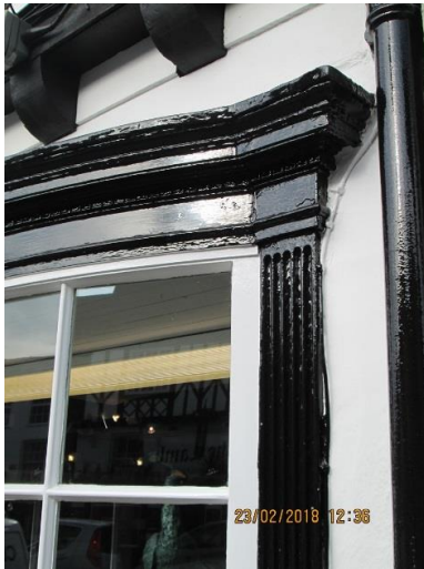
Left: Detail of a typical shop front of the period before c.1850 (51 Market Street, Ashby de la Zouch). A fluted pilaster with capital supports a shallow classical frieze and cornice. Note the absence of a bracket. The shop window is bowed and divided into small panes.
