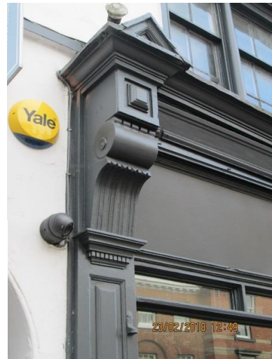
Right: Detail of a typical shop front of the period after c.1850 (76 Market Street, Ashby de la Zouch). A panelled pilaster supports a deep canted fascia and cornice. The fascia is bounded by a bracket. The shop window is flat and contains plate glass; note the narrow overlight.
