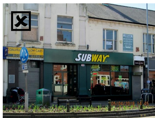
6 Marlborough Square, Coalville. The shop front fails to respect the ‘original division’.
