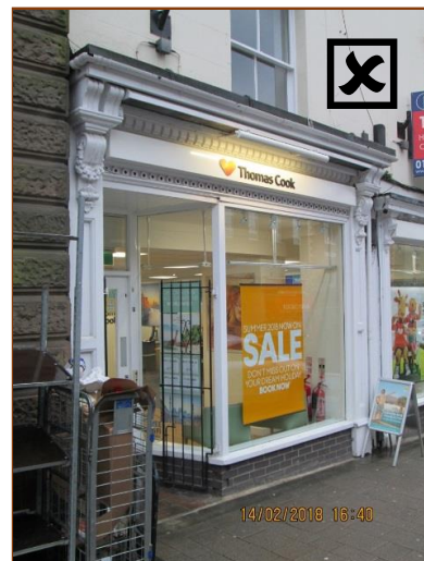
72 Market Street, Ashby. Poor signage devalues this nineteenth century shop front.
