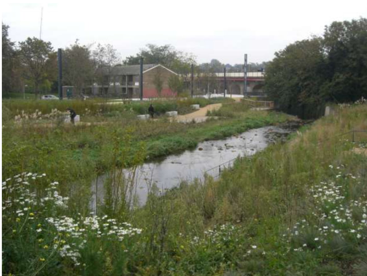
River Quaggy, Lewisham restored from culverting and naturalized improving biodiversity, access to nature and flood prevention
