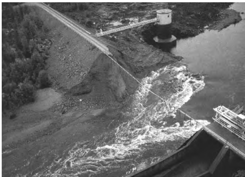
Breach of Noppikoski Dam, Sweden, 1985
