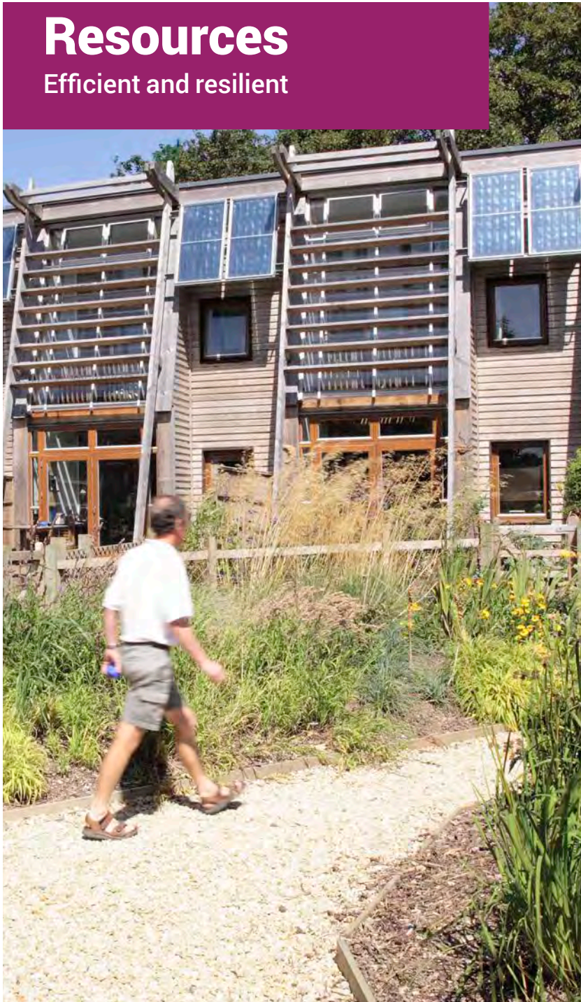
Low energy housing with passive solar design, including shading to prevent overheating in summer, and highly insulated thermal mass construction. Great Bow Yard, Langport, Somerset
