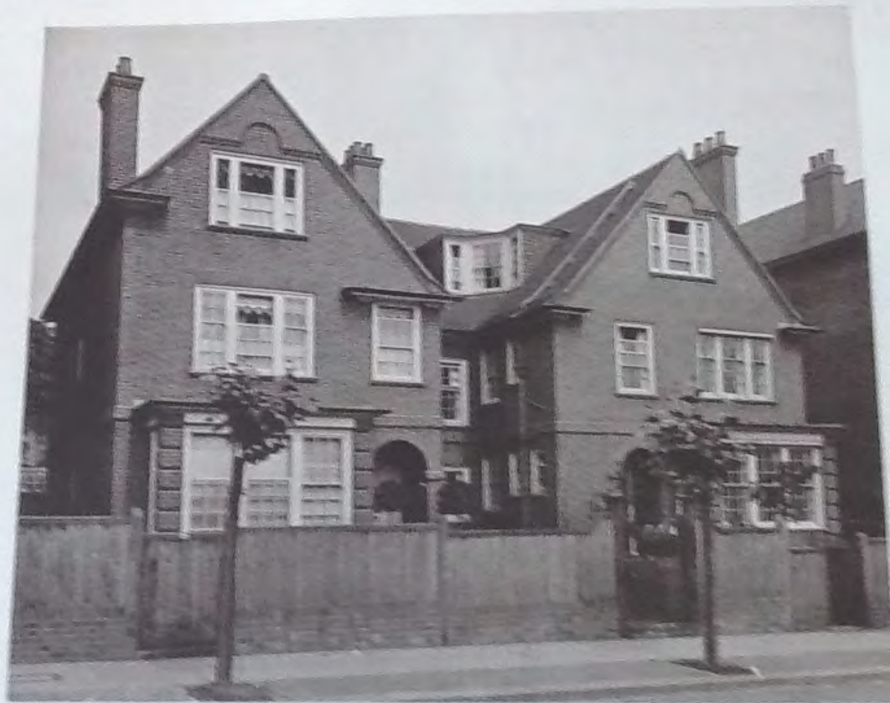
House No. 12, Central Avenue
