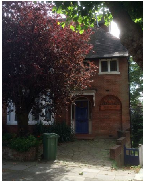
FRONT VIEW OF 16 HOLLYCROFT AVENUE, LONDON NW3 7QL
