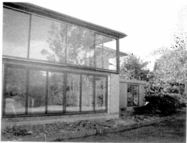
7. First floor glazing in photograph attached show example of powder coated fine line window frames
