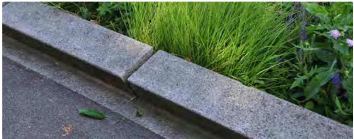
Broken kerb detail for bioretention
