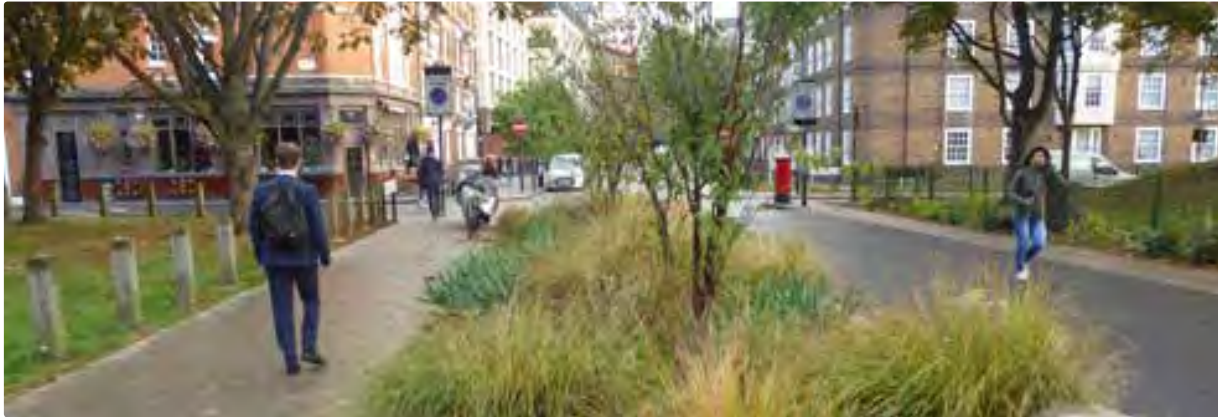
Bioretention rain garden in Vauxhall
