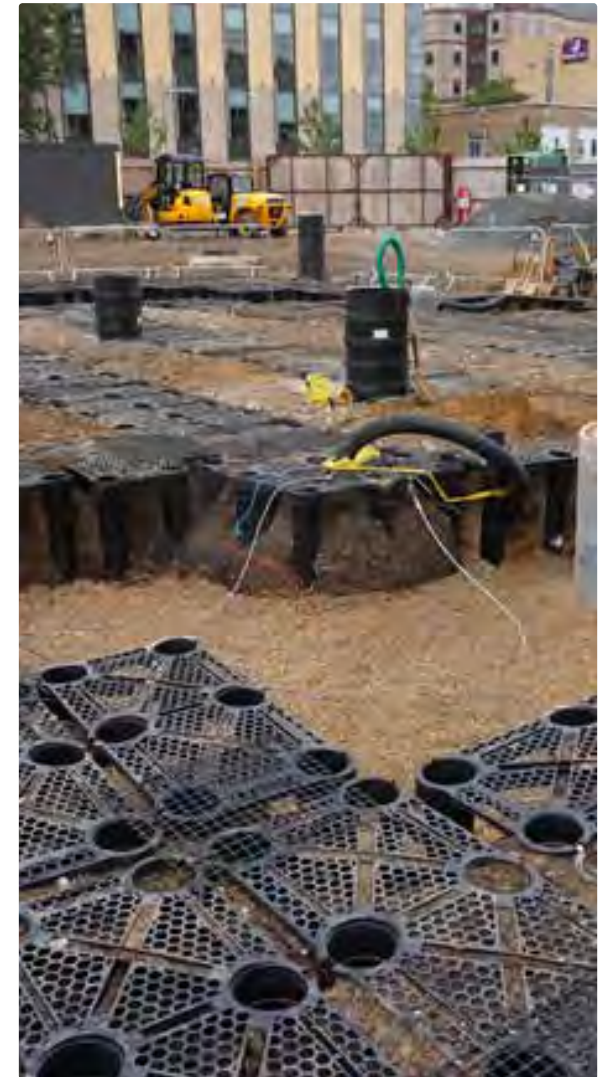
Attenuation: soil cells
