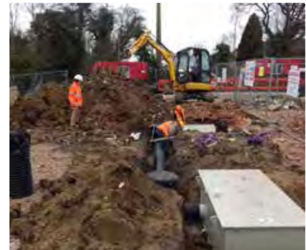
400m 2 swale under construction
