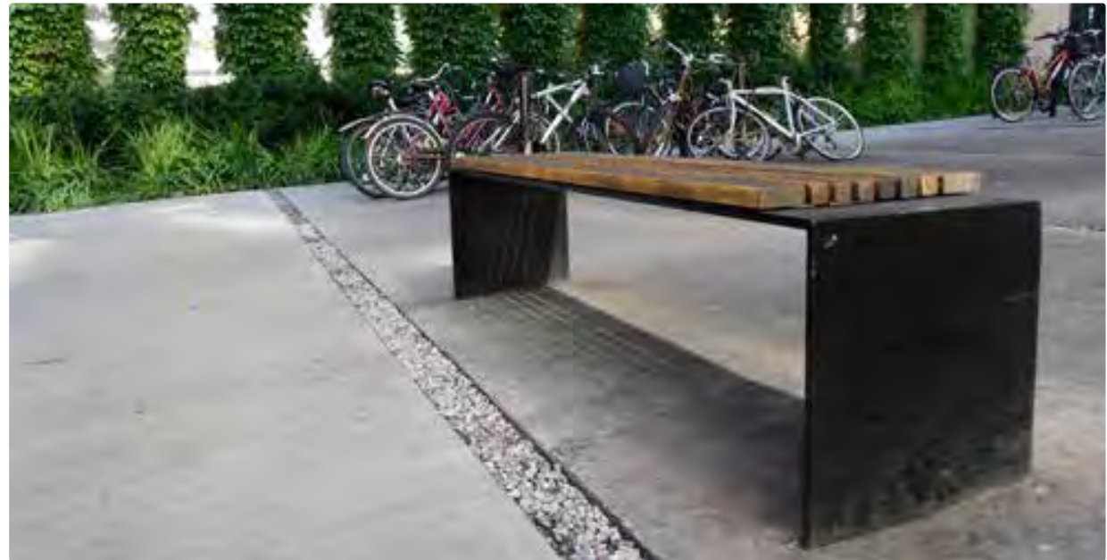
Filter drain: open gravel filled joint
