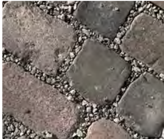
Quantity: permeable paving, grit jointing
