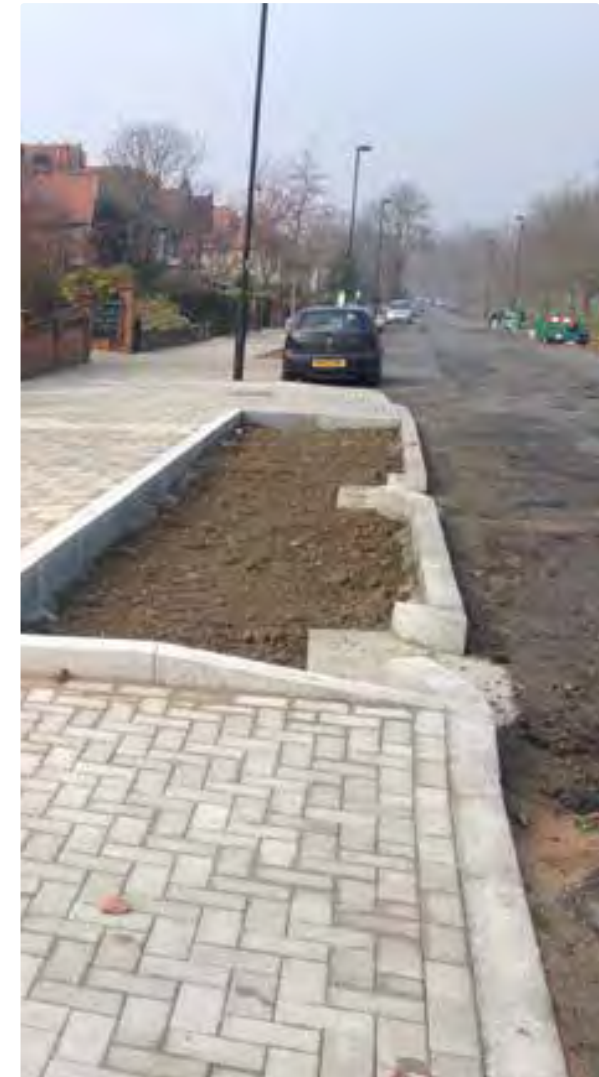
Kerb inlet and de-pave detail
