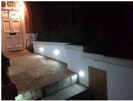
Photo BGI 5: Motion Sensor Lighting, Illuminating Specific Areas Only When Needed
