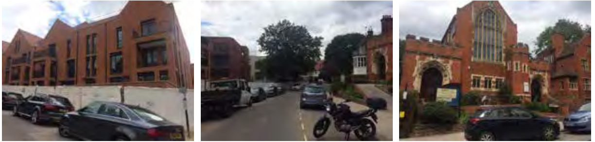
Kidderpore Avenue: excessive bulk and massing of new development opposite Grade II listed church and adjacent to Arts and Crafts houses
