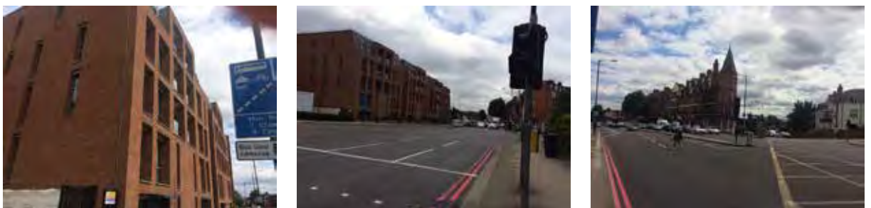
Finchley Road: excessive bulk and massing of new development opposite Grade II listed banking hall and adjacent to Arts and Crafts houses
