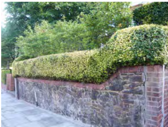
Photo BGI 2: Front Garden Hedge and Retaining Wall, Bracknell Gardens, Sub Area 6
