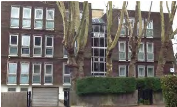
Photo DS 4: 27 Redington Gardens, Front Elevation
