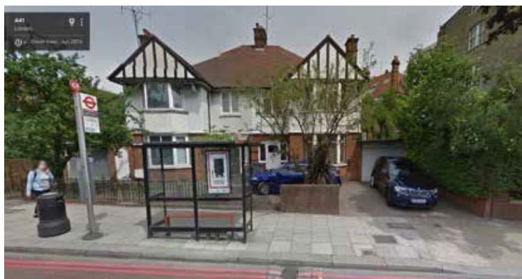
Photo DS 20: 282-284 Finchley Road, Streetscape
